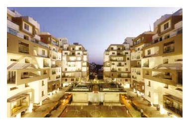
daylight and natural ventilation into its design. Fly ash bricks were used during construction and a significant portion of the building has been devoted to vegetation to reduce the urban heat effect. The building also integrates wastewater recycling and solar energy among its green features.
